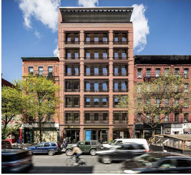
The Charlotte's air-filtration and passive-home construction added an estimated 15% to building costs. PHOTO: CHRISTOPHER PAYNE/ESTO
